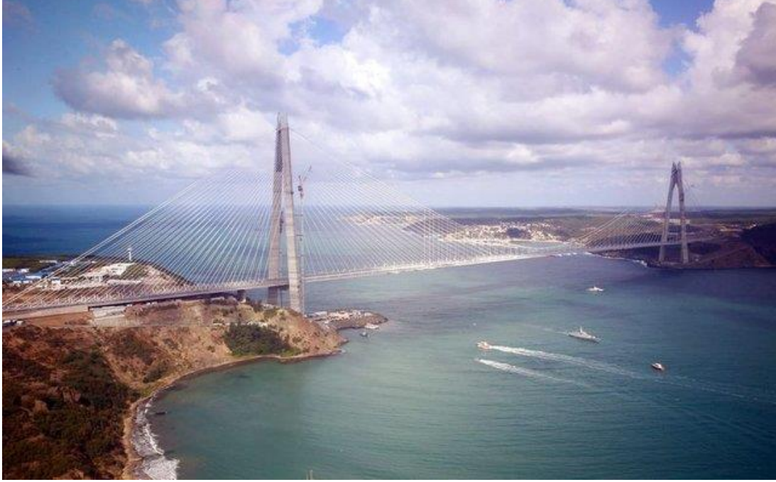
Image 10 Yavuz Sultan Selim Bridge / 3. Bridge 17
